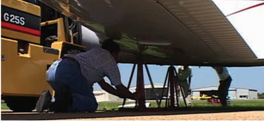
Place main jacks under the jack points as soon as the airplane is high enough. Now it's solid.
